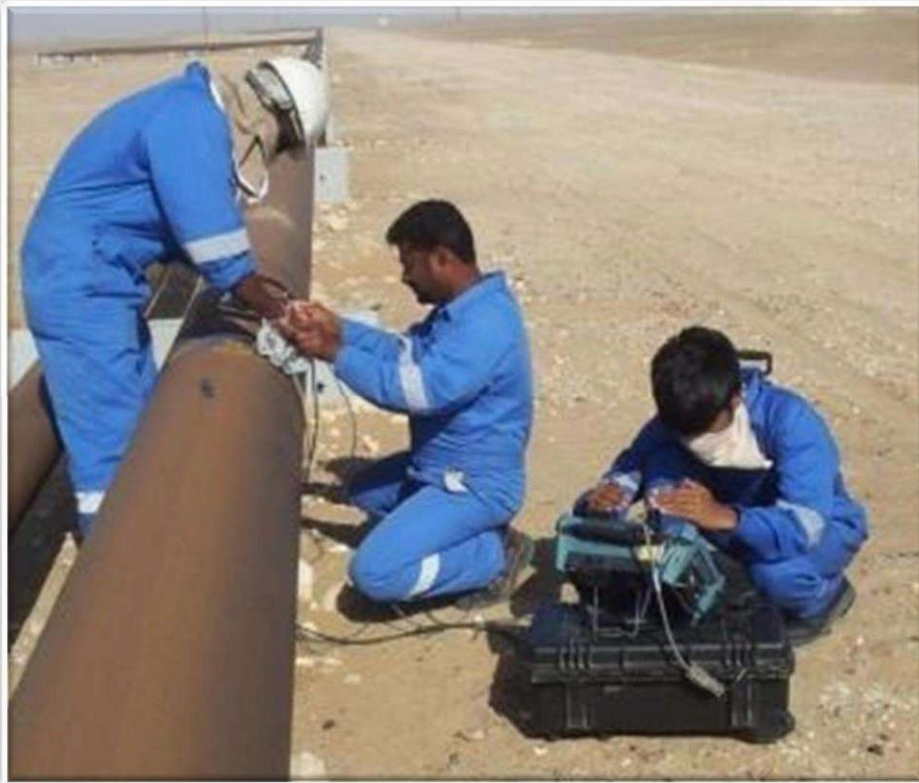
PAUT Inspection Of Pipelines for PDO Oman
