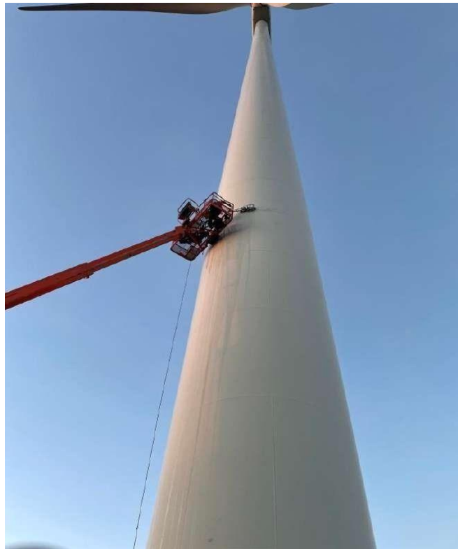
Inservice Inspection of windmill Tower Using SteerRover for SGRE in Bijapur, India
