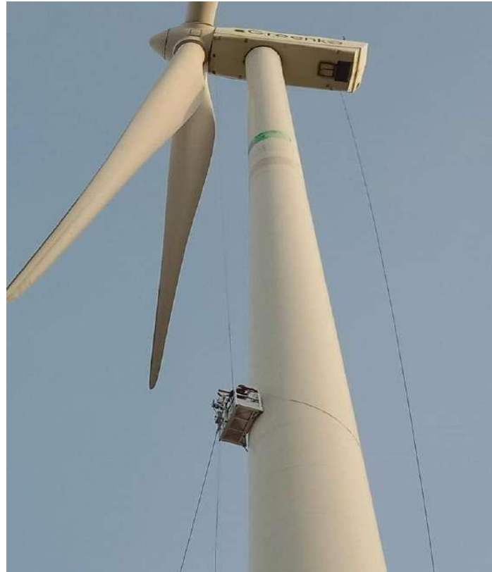
PAUT Inspection of Windmill Tower using Tower supporting platform for Siemens Gamesa
