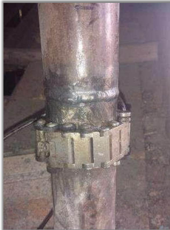
PAUT of Power Plant Piping Using Cobra Scanner at Sonichar, NIGER
