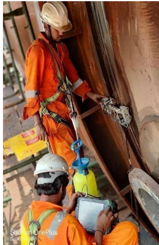
PAUT & TOFD Inspection of CDU & VDU FORLTHE at IOCL Barauni, India
