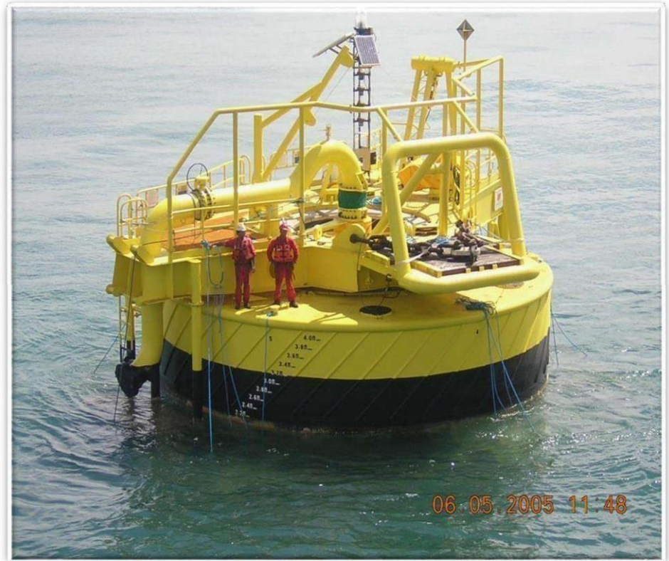
SBM Installation Inspection - Ghana
