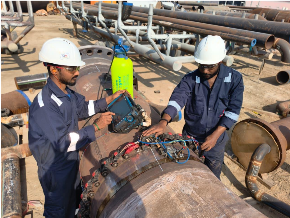
PAUT Inspection of Piping Joints at MS SHAW, UAE (Abu Dhabi National Oil Company)
